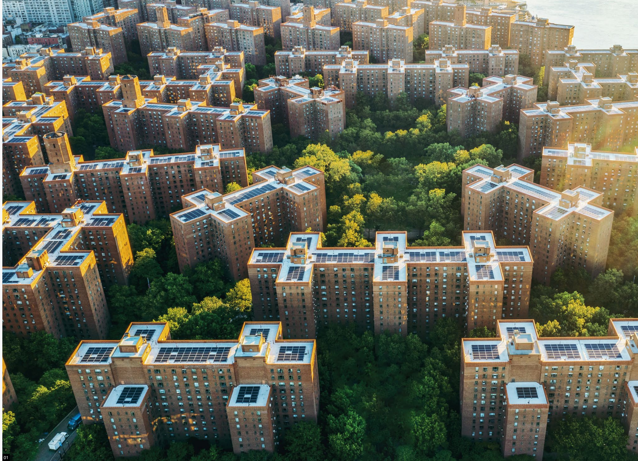
— 01 Rooftop solar across Blackstone's multifamily residential asset, StuyTown
